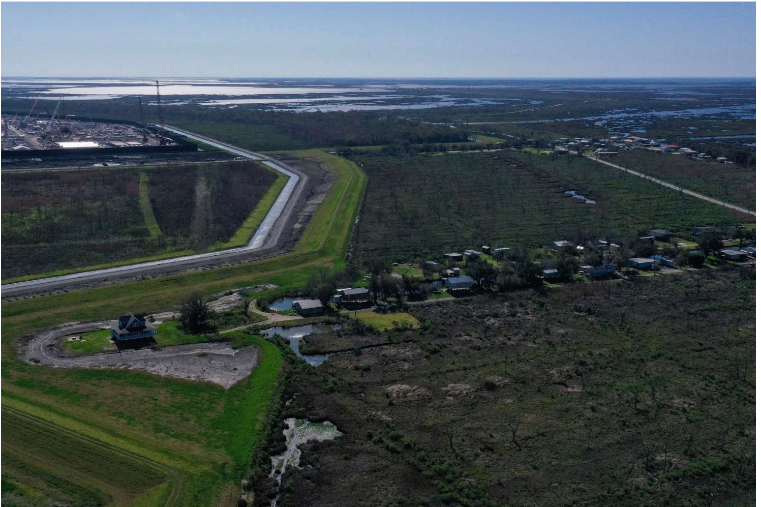
A small community of houses along a canal next to Plaquemines LNG.
