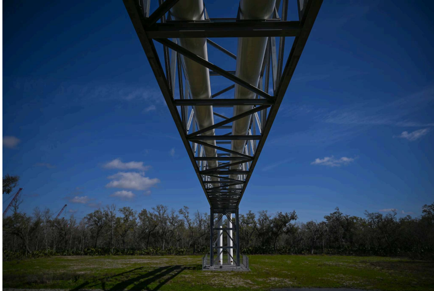
Pipelines raised above the levee system surrounding Venture Global's facility.
